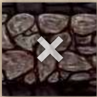
Wall of stone
